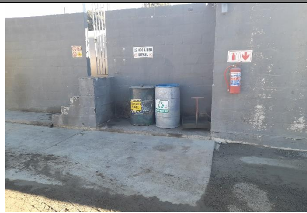
Hazardous waste bins fitted with lids
