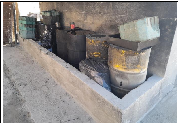
Hazardous waste storage area
